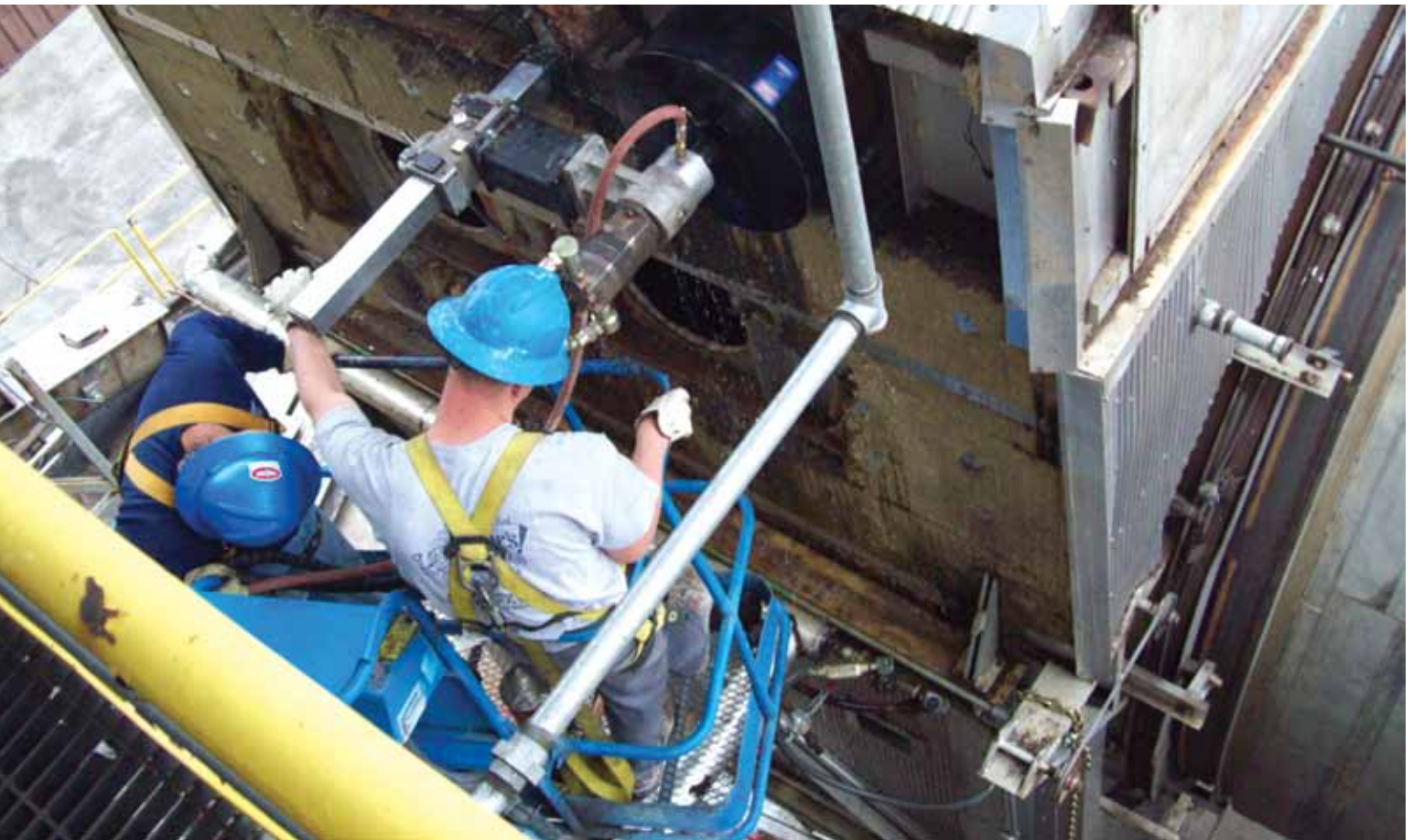
The contractors carefully maintained drilling speed and pressure to achieve success.
