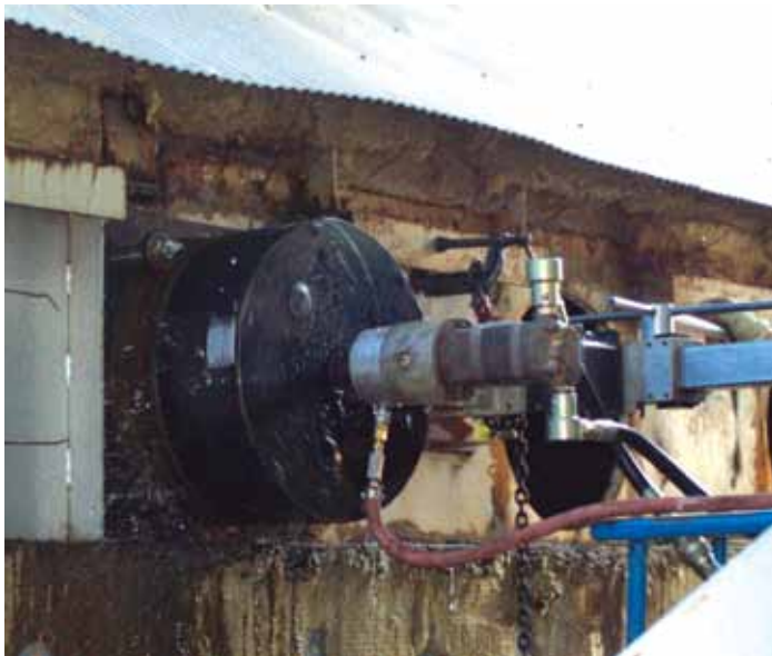
Nine 20-inch diameter holes were drilled by Taylor's.
